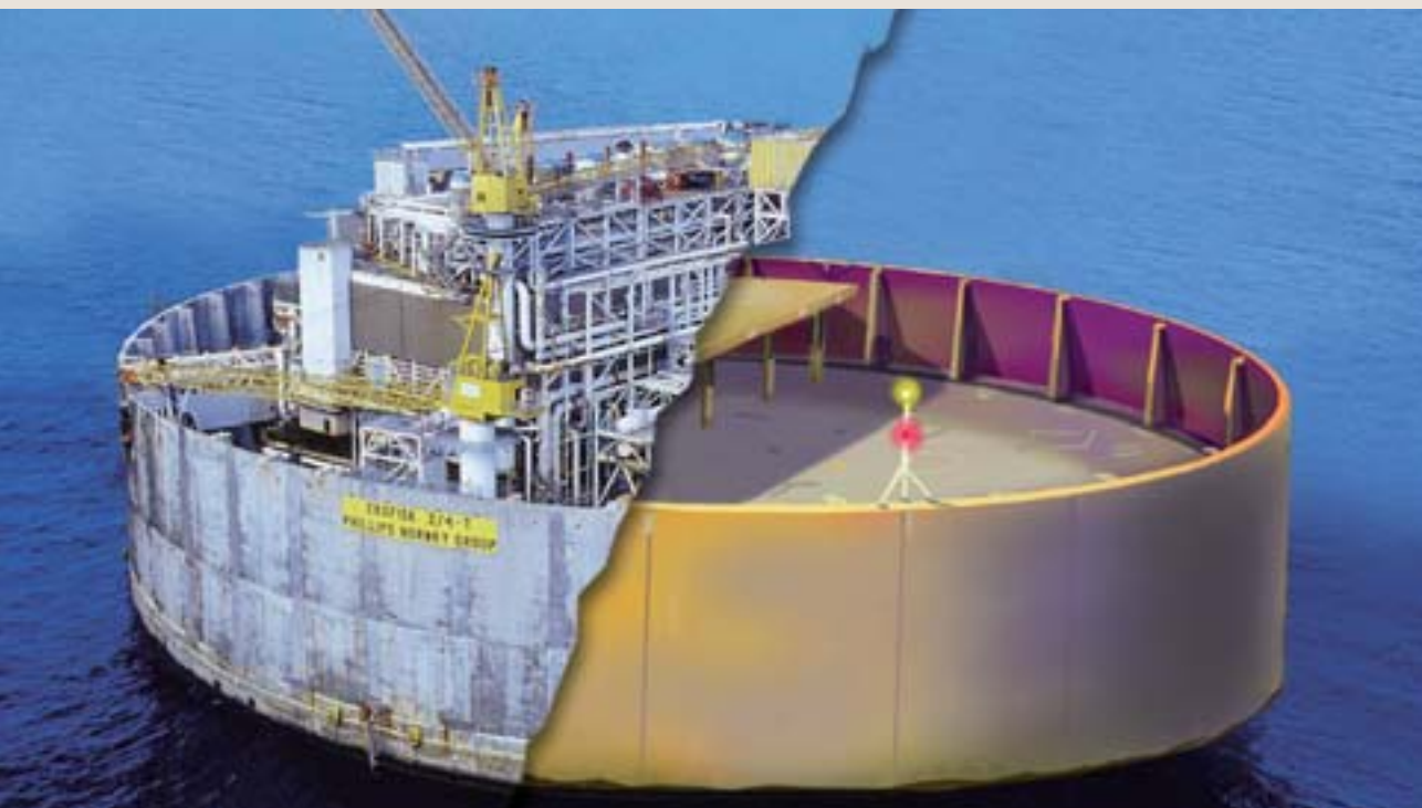
Figure 7.2 Illustration of the Ekofisk Tank, before and after removal of the superstructure (Source: ConocoPhillips)
